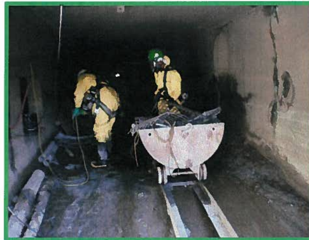
Repair Damaged Areas
