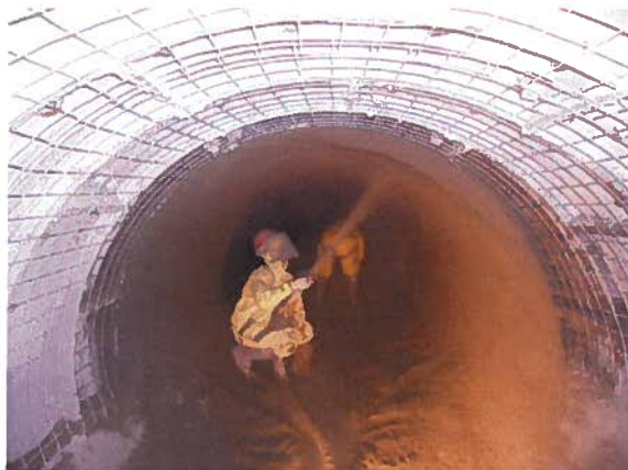
Spray-on Surface Coating
