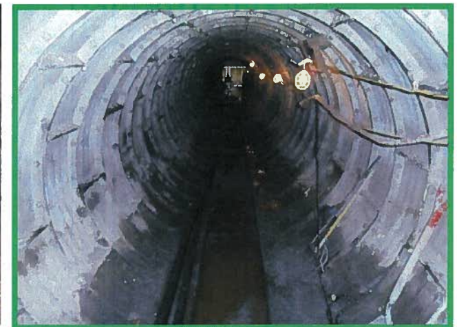
Grouting Seals Plates
