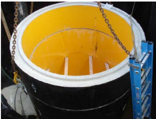
Installation of manhole at 15 th Street storm drain
