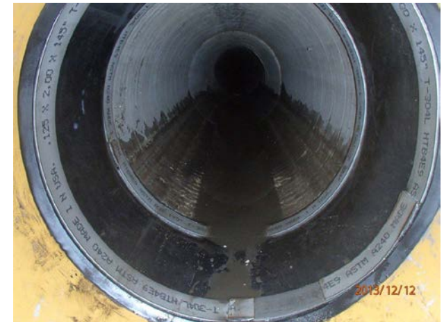
15 th street storm drain relining in progress
