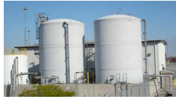
A storage tank will be added to existing tanks
