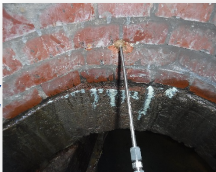
Structure grout injection prior to relining
