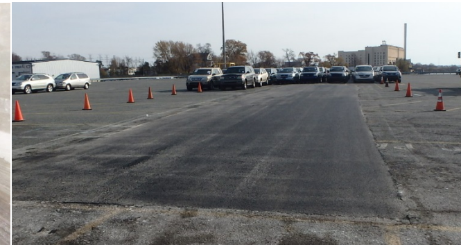
Asphalt surface cover being placed at location in Area 1600
