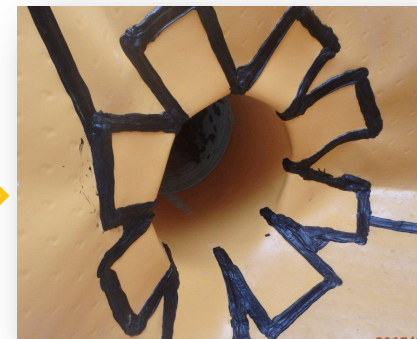
Transition strip from lined pipe to inlet
