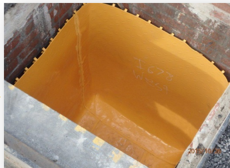
Inlet relining in progress
