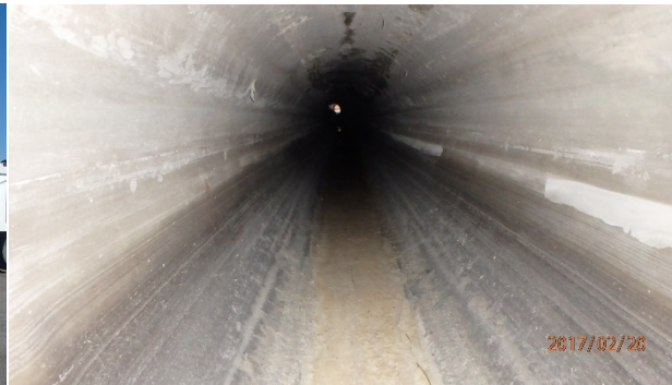
Lined 12 th Street Trunk Line
