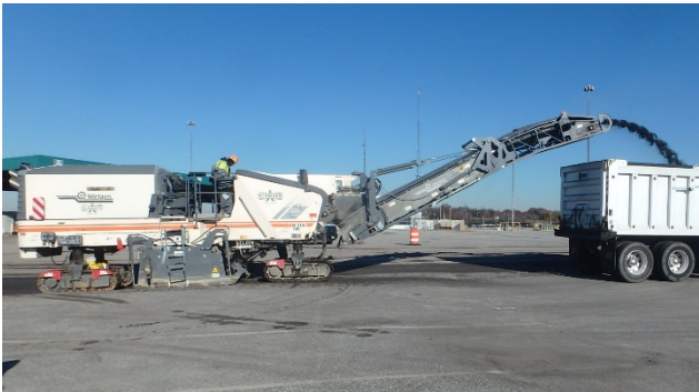
Asphalt milling in Area 1600
