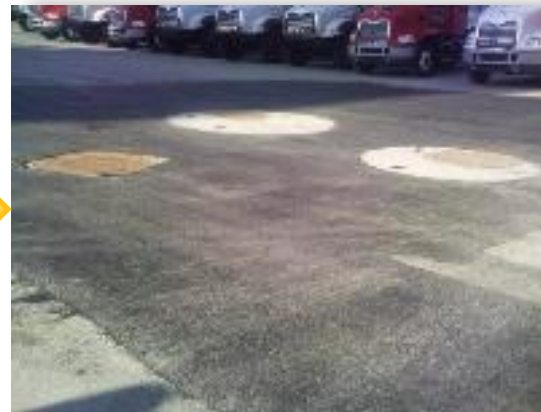
Transition strip from lined pipe to inlet
