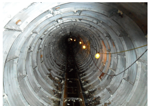
Metal plates inside of storm drain prior to relining activities; over two miles of storm drains have been relined to date
