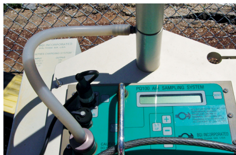
Monitor measures air at work zones and perimeter of Terminal
