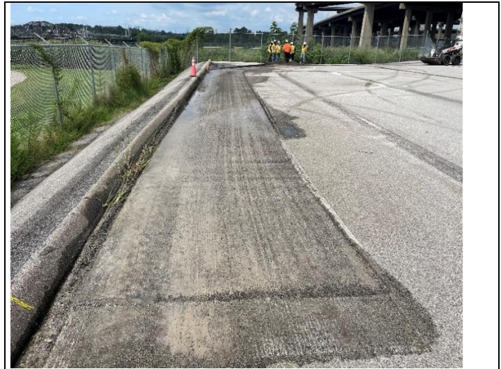
PHOTO 6 Milled drainage channel
