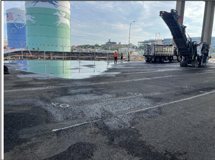
PHOTO 1 Survey mark out for milling and paving
