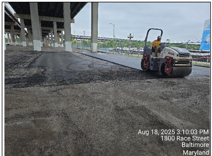
PHOTO 8 Vibratory roller compacting surface course asphalt
