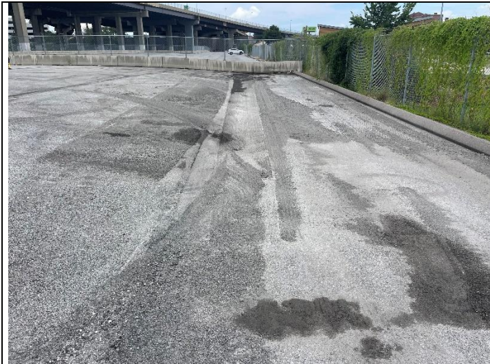
PHOTO 5 Milled drainage channel
