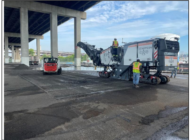
PHOTO 2 Asphalt removal using milling machine
