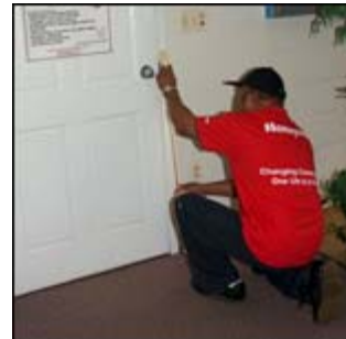
On April 26, Honeywell volunteers partnered with Rebuilding
